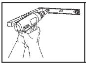
**13.** Position the Bracket over the holes or anchors. Screw in the 3/8" lag screws. A combination of lag screws and wall anchor can be used.
